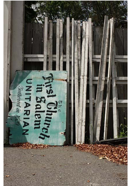
Images of clean up and preparation for renovation.
